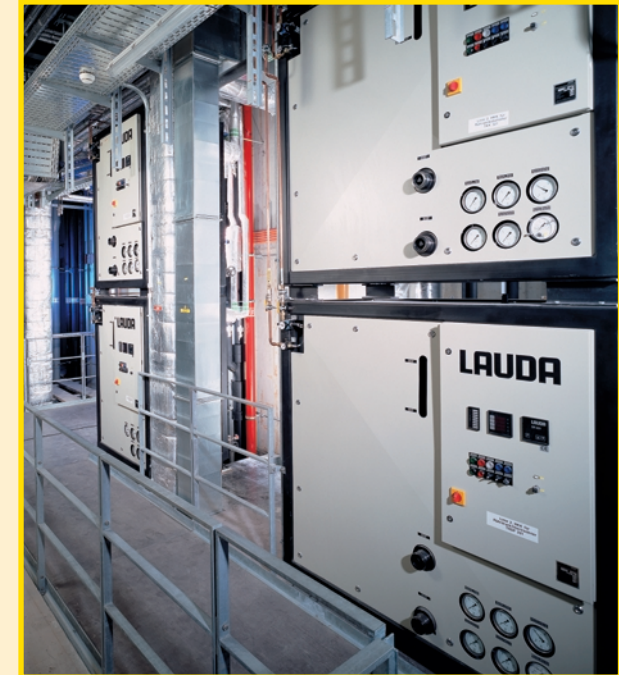
Module construction of the secondary circuit units
