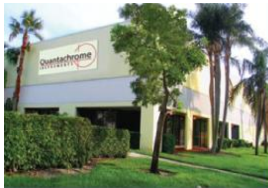
Quantachrome Instruments' corporate headquarters in Boynton Beach, Florida.
