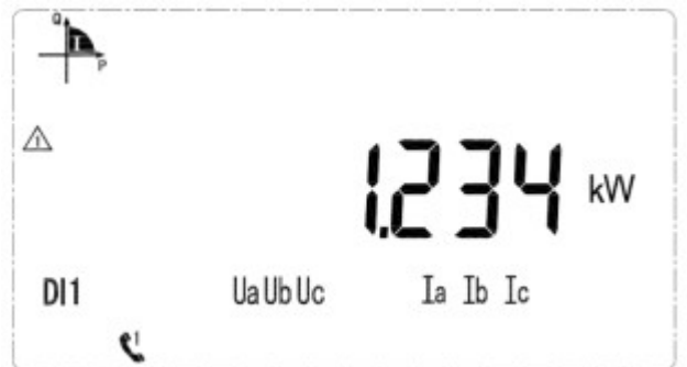
Current total power is 1.234kW
