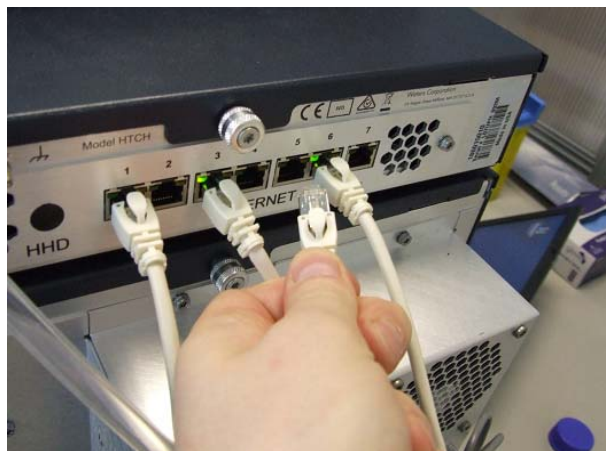
Figure 12 - Router for ACQUITY UPLC connections
