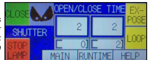
601-series touchscreen power supply automatic shutter control screen
