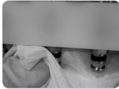
1. Remove old grease.
